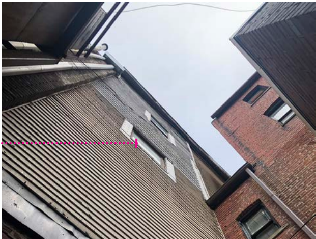
VIEW OF ADJACENT WINDOWS TO NORTH
