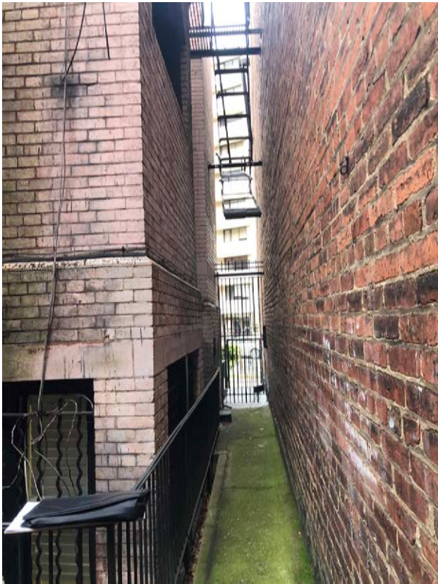
FROM REAR COURTYARD LOOKING TO 18TH STREET
