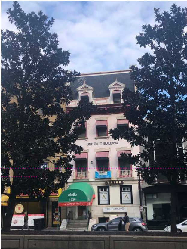
BUILDING TO NORTHWEST
