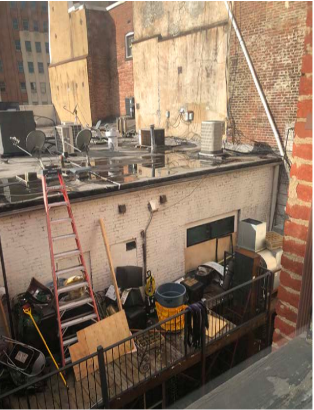
VIEW OF ADJACENT BUILDING TO WEST
