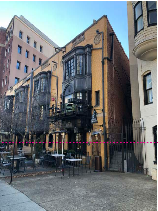
BUILDING TO SOUTH
